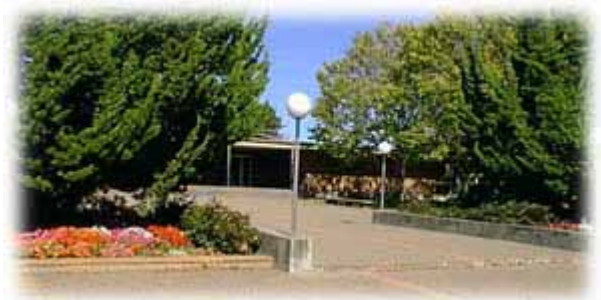
Complex Litigation Courthouse San Mateo, CA
